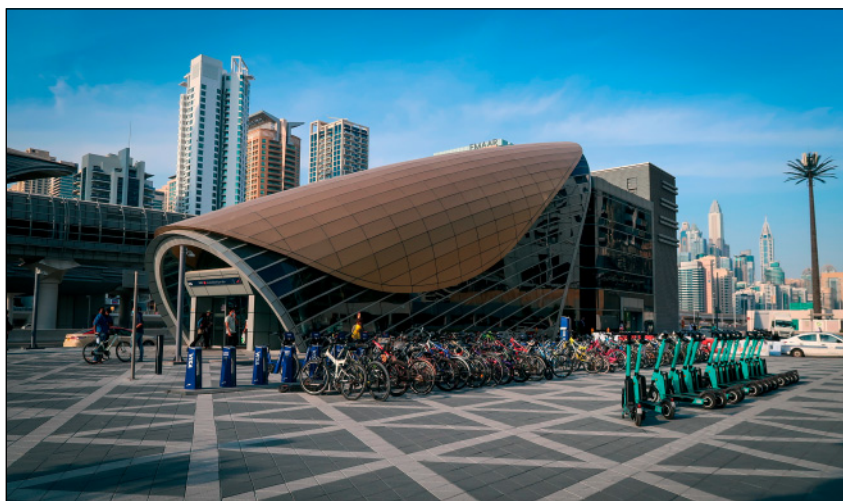
Stanice metra DMCC
