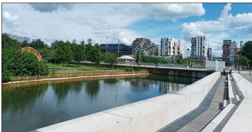
Hydraulic tank at Docks de Saint-Ouen
